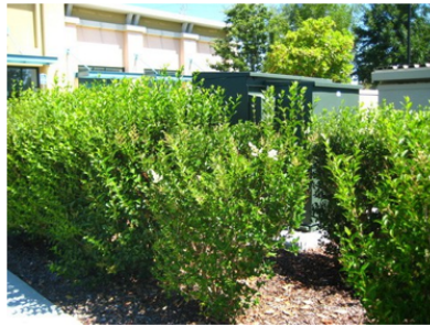
Exterior utility equipment screened with planting
