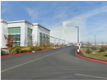
Utilize Planting Islands with Large Trees and Shrubs at Truck Court Entrances
