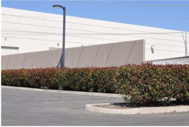
Use of wing walls and landscaping to conceal loading docks, and service doors
